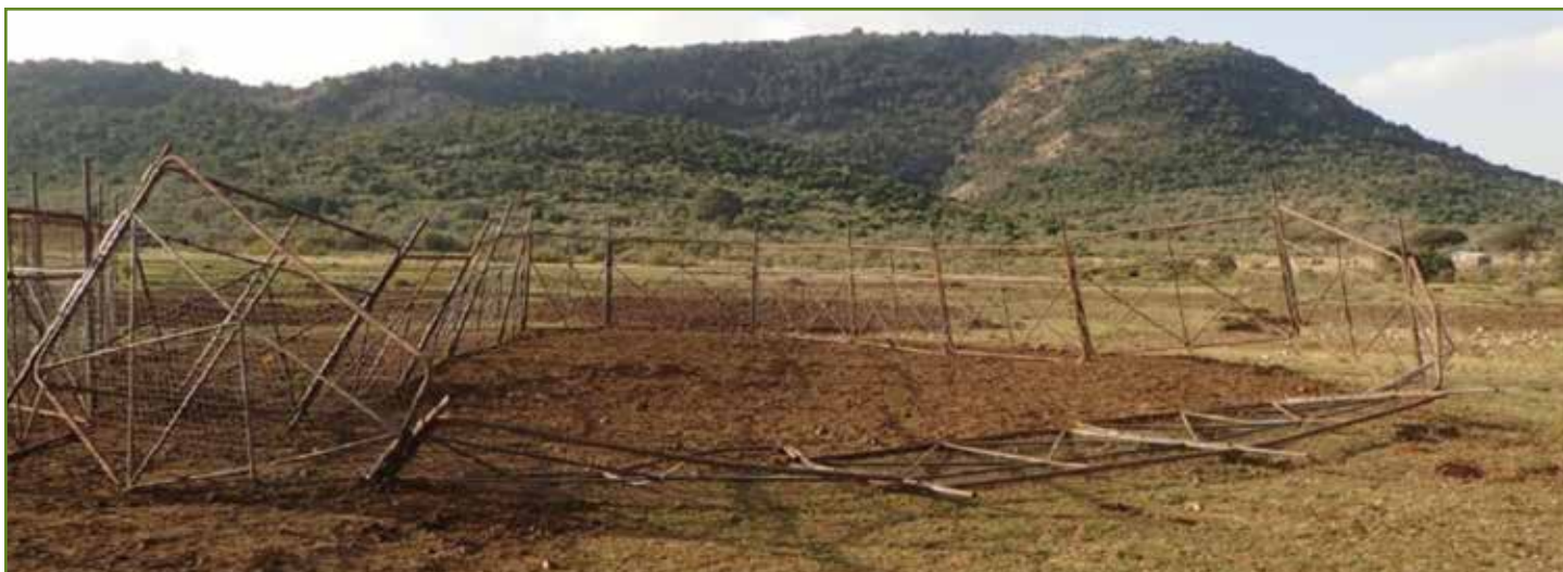
Mobile bomas, if not constructed properly, are vulnerable to being knocked down by frightened cattle. Proper construction of these bomas is critical for animal safety.
